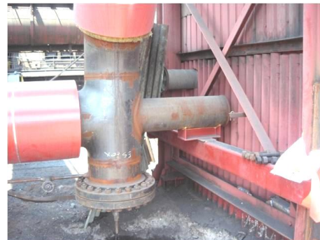
Figure 8-4: Drip Leg with Flanges
